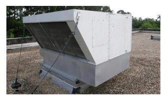
chillers produce cold water, which is pumped to one or more air handlers or fan coil units throughout the building, where the water absorbs heat from warm indoor air. The cool air is then distributed around the building through a network of ducts. Water-cooled chillers, which use a cooling tower to remove heat, are typically more efficient than aircooled chillers, which blow air across the condenser coil.
